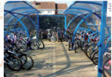
Cycle parking at Parlaunt Park Primary School For further information please visit: www.sustrans.org.uk/slsat
